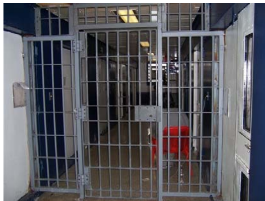
Corridor breaker-gate creates “dayroom”
